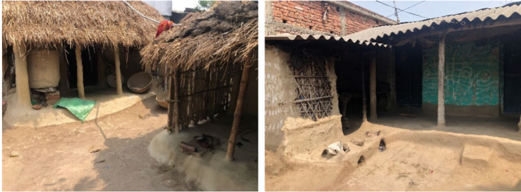
Fig. 8.1 Typical kutcha houses in Bahuarwa, made of mud, bamboo, and thatch (left), and gradual transformation into a pukka house (right) (Authors 2022)
